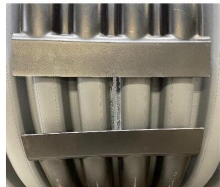
2. Once the bottom half of the coupler is in place, place the second half of the coupler over the top the spliced pipe so that it aligns with the bottom half of the pipe. Again, this will sit evenly between the two halves of pipe, with the splice in the middle and two corrugations of each half.
