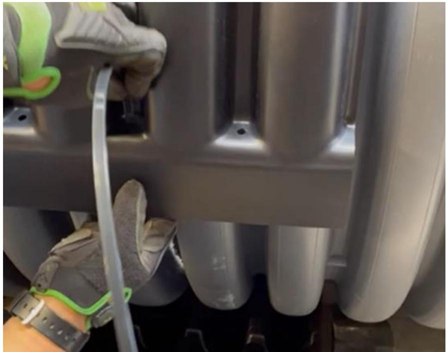
b. Continuing to thread the zip tie through until you have enough slack to thread through the second middle hole located on the other half of the coupler. Note: this will go through the inner hole of the second half of coupler, not the outside.
