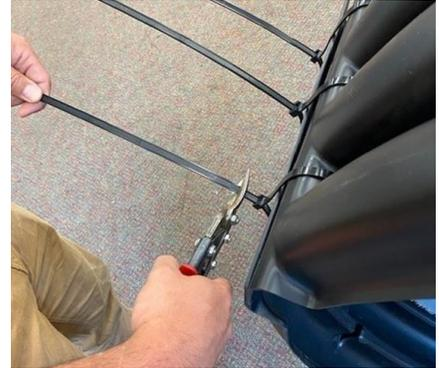
10. After the six zip ties have been zipped tight and ends have been trimmed, the split coupler has been installed.
