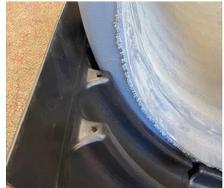
4. Once both halves of the coupler are centered around the pipe and the zip ties holes are aligned, the included zip ties can be used to secure the coupler to the pipe. The best practice to thread the zip ties through is to first thread a zip tie through the middle hole on both ends of the coupler. Start with one side, cinch the zip tie, and move to the other side and repeat the process.
